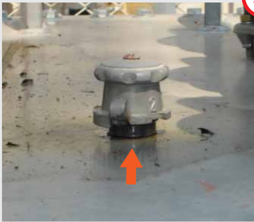
Oil Leakage at Gasket
