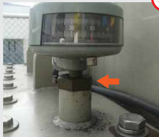
Oil Leakage
