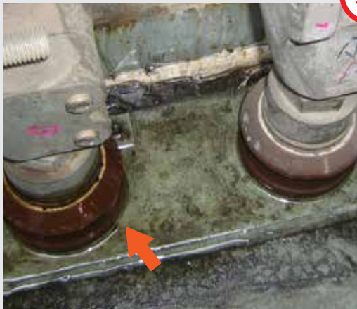
Oil Leakage at Gasket
