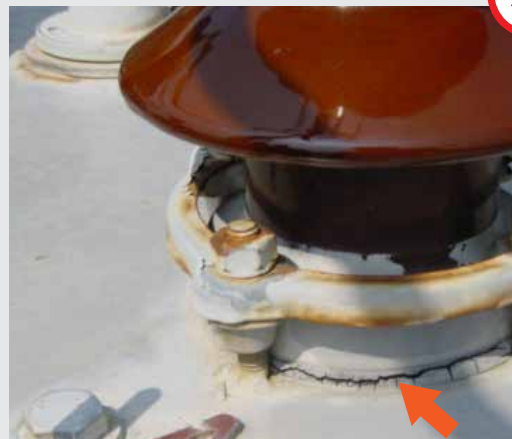
Deteriorated Gasket
