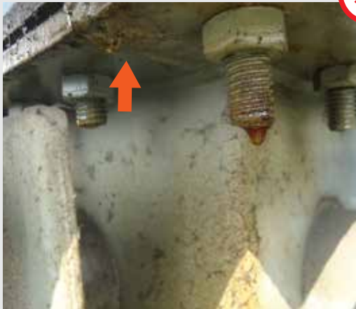
Oil Leakage at Gasket
