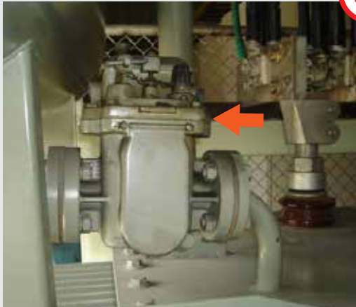
Oil Leakage
