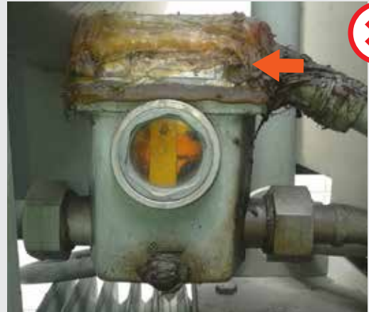
Oil Leakage
