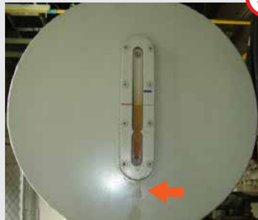
Leakage at Conservator Tank of Open Type Transformer
