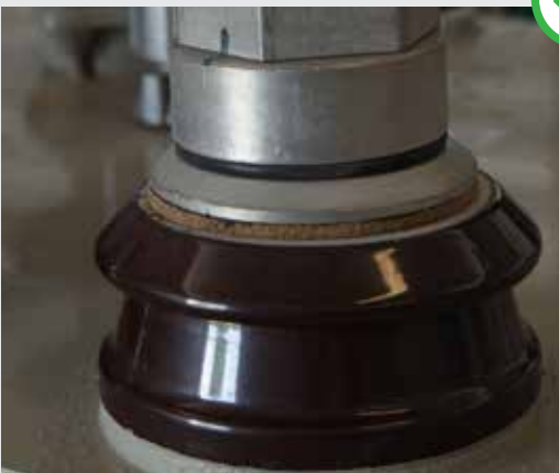
Complete LV Bushing Gasket
