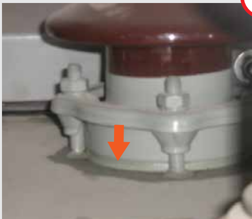
Oil Leakage at Gasket
