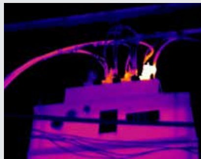
Photo of heat at LV Terminal
