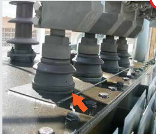
Deteriorated Gasket
