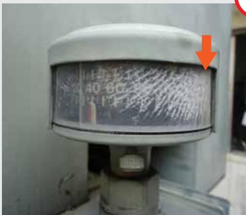
Cracked at Dial Window
