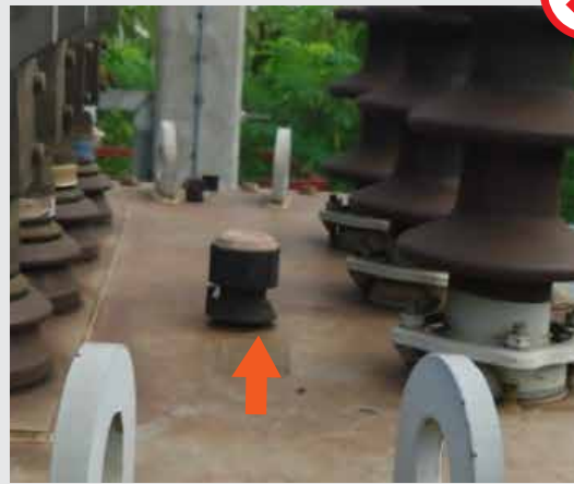
Deteriorated Gasket
