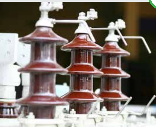
Complete HV Bushing
